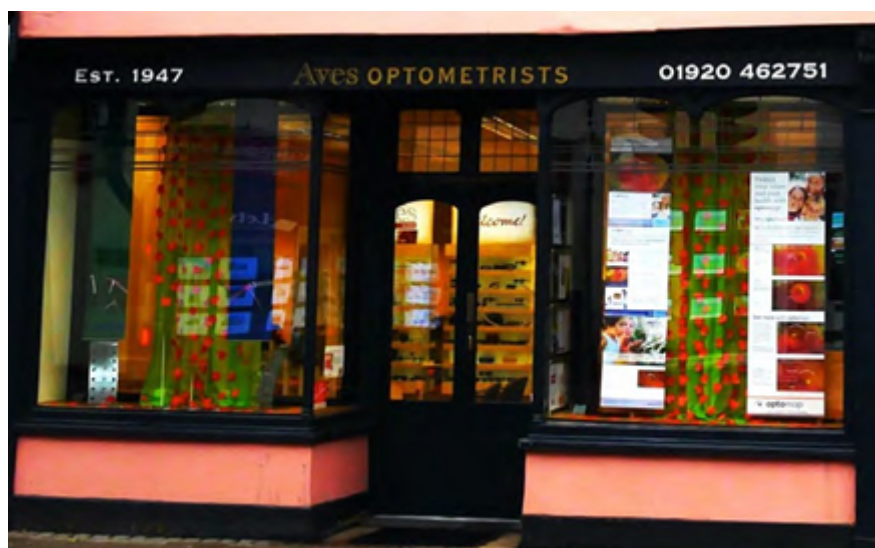
Figure 36- Appropriately scaled lettering to height of fascia.
