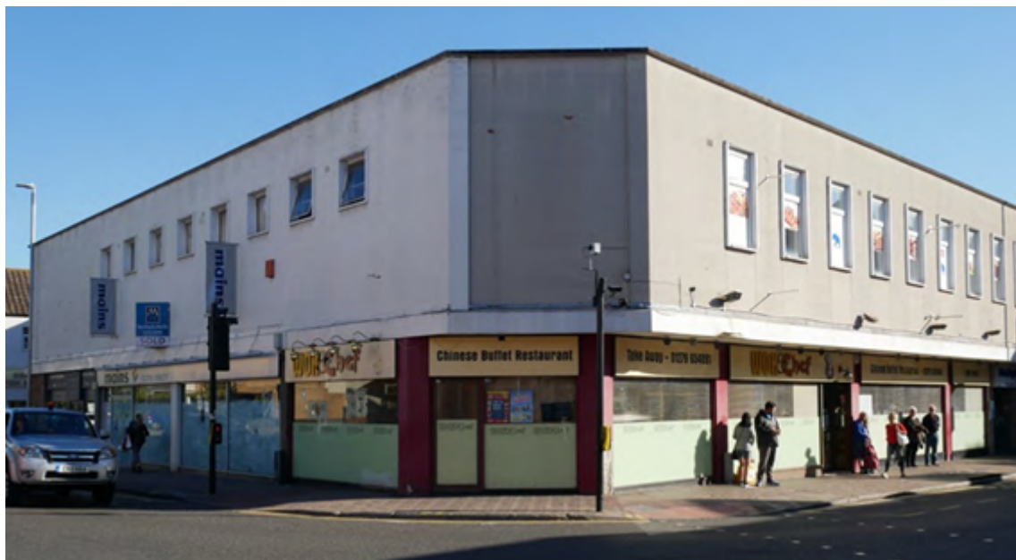
Figure 10 – A less than successful 1960's parade of shops on the corner of South Street & Station Road.
