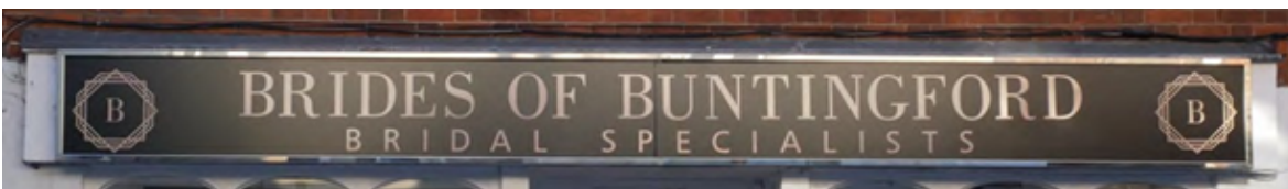
c) Although easy to read, the lettering is too large and thus crowds the applied fascia board. A hand-painted fascia would have been more successful.
