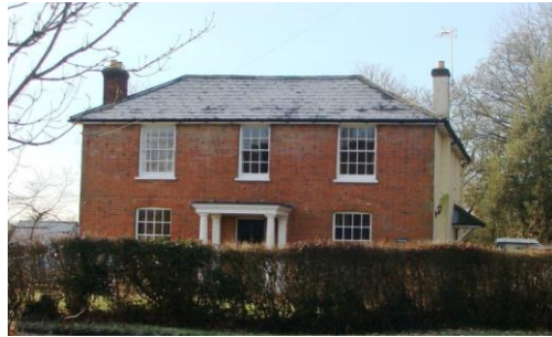
Picture 16. The Hale - makes a worthwhile architectural and historic contribution to the conservation area in this location.
