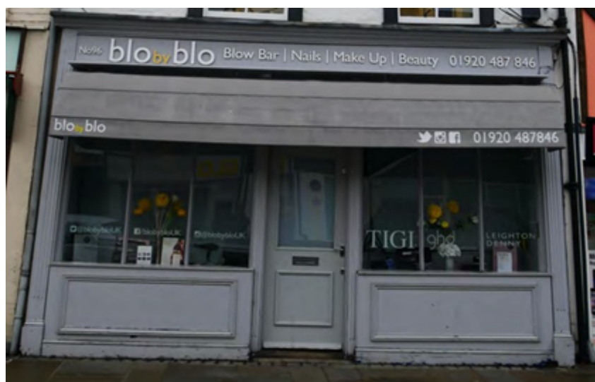
Figure 37 – Example of a fascia with a too much lettering and an inappropriate Dutch blind.
