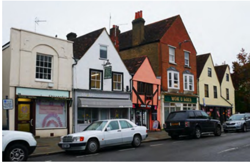
Figure 5 - A variety of architectural styles, some inappropriate shopfronts and blinds
