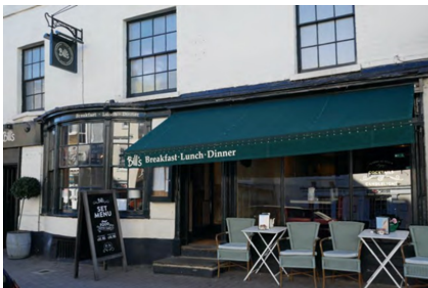
Figure 45 – An historic shopfront that could not accommodate access for the less able without significant harm.
