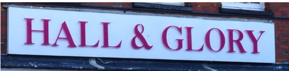
e) An inappropriately positioned plastic board placed above the ground floor with large lettering. An uncomfortable relationship.
