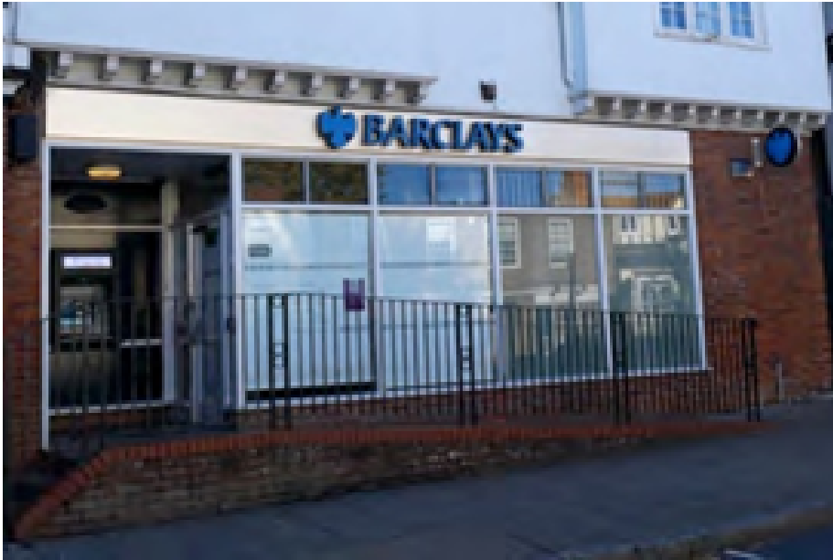
Figure 48 - Both the ramp and shopfront make for an unacceptable impact on the building and streetscene
