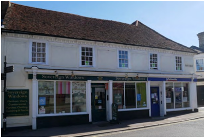
Figure 16 - Early 18th century frontage to a 16th - 17th century building. Generally retaining traditional details but with some modern signage and swan neck lighting.
