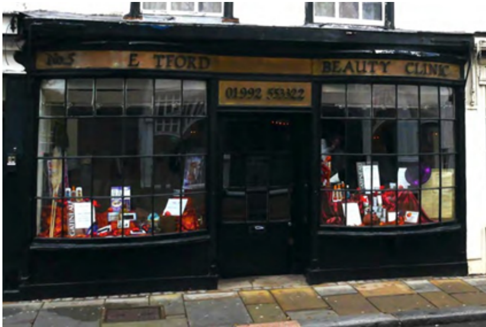
Figure 17 - Early 19th century frontage, double fronted with multi-paned oriel bays including slim glazing bars and traditional features.
